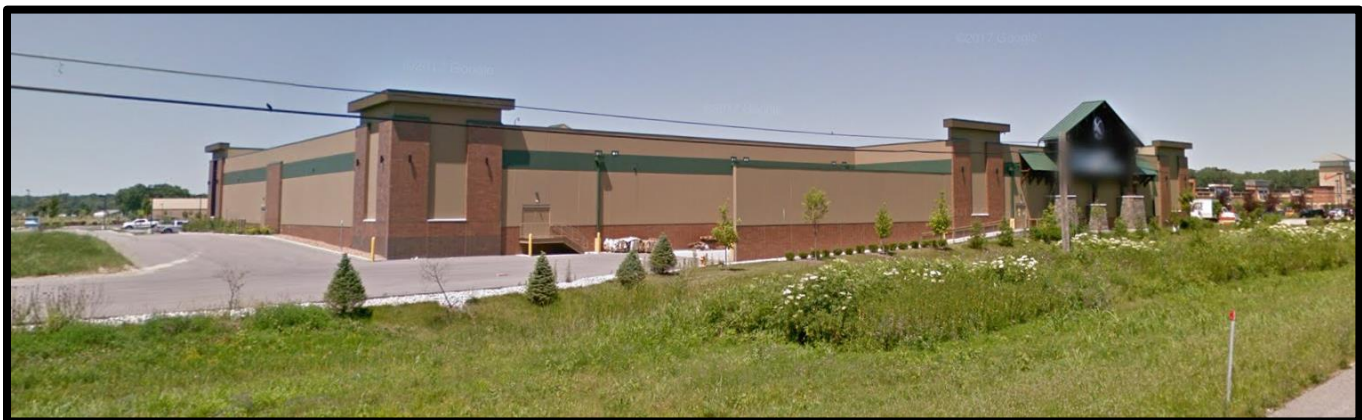
Figure 6: Loading dock with screen wall
