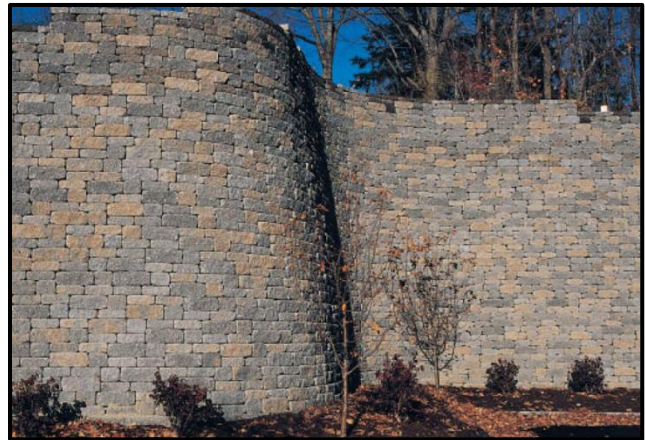
Figure 7: Mosaic Retaining Wall
