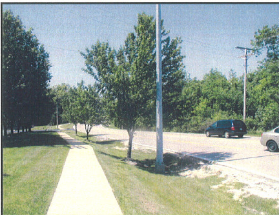
Northern view along Wilson Road
