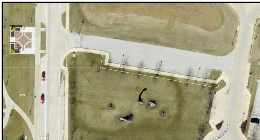
Figure 7: Existing parking area on south side of subject property
