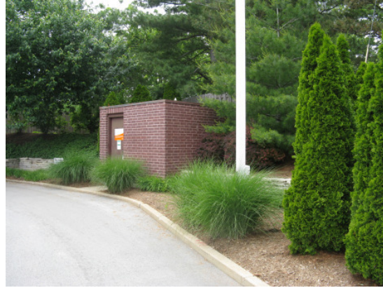
Existing Equipment Compound
