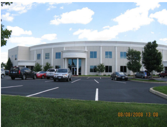
View looking southeast at the site
