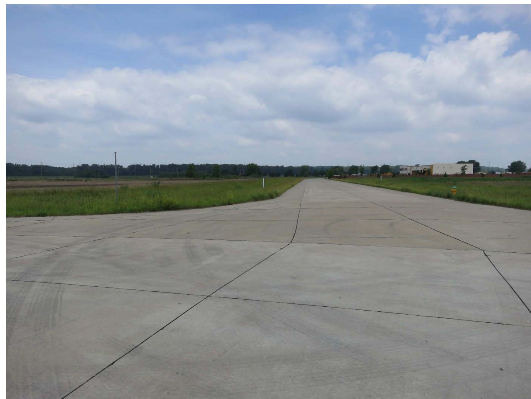
A - VIEW LOOKING NORTH
