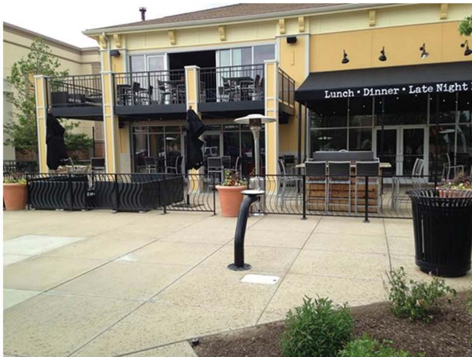
PATIO STRING LIGHT UNDER FABRIC AWNING (RIGHT HAND SIDE)
