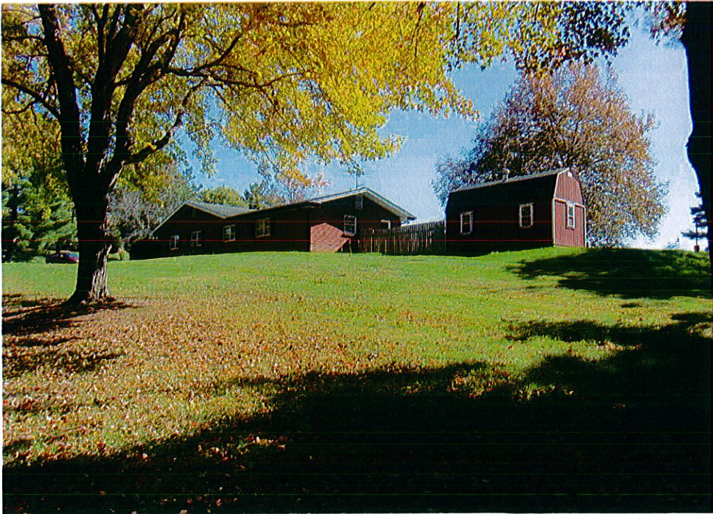
LOOKING NORTHEAST AT BACK OF HOUSE FROM BACK YARD
