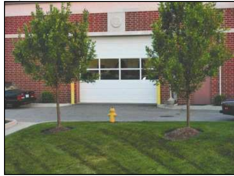
Bentley Shop Garage doors from US 40/64
