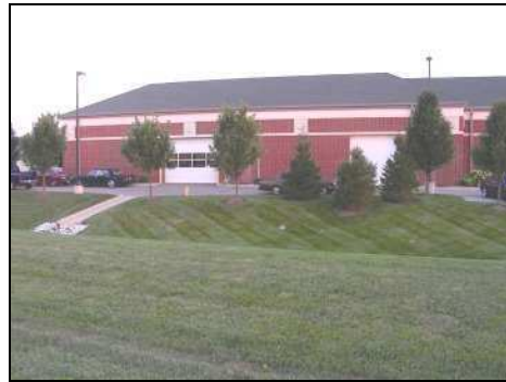
Bentley Shop Garage doors from US 40/64
