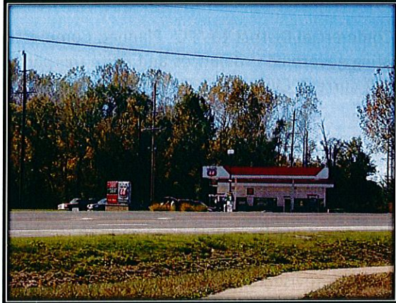
Existing Service Station—View from North Side of Chesterfield Airport Road
