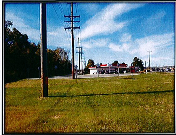
Existing Service Station—View from Eastern Property Line
