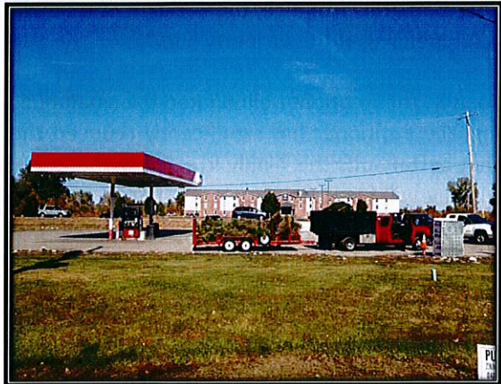
Existing Service Station Canopy—View from Old Olive Street Road
