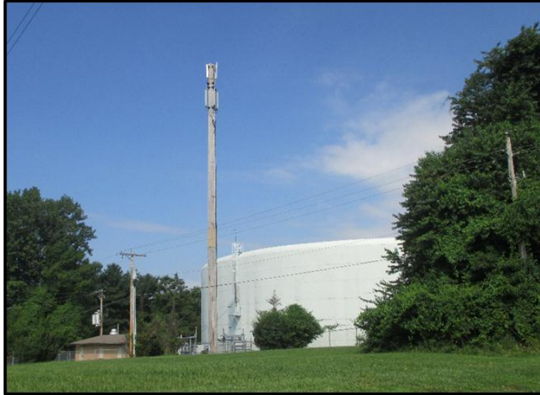
Figure 2. Site Photo – North and East Facades
