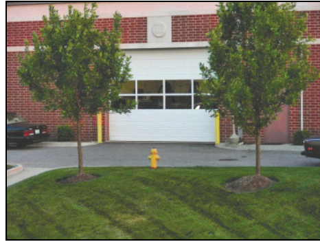
Bentley Shop Garage doors from US 40/64
