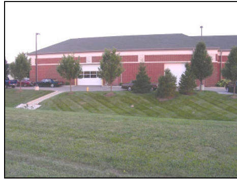
Bentley Shop Garage doors from US 40/64
