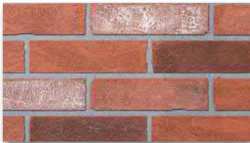
Used Wall Brick
