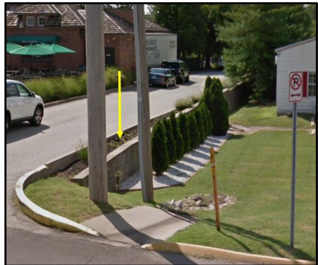
Figure 5: Existing Retaining Wall
