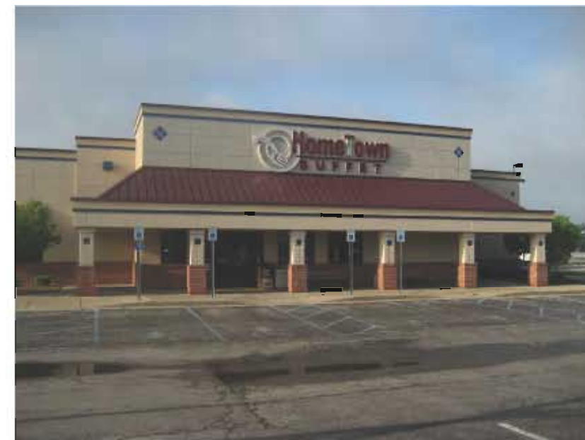
NORTH VIEW OF EXISTING BUILDING
