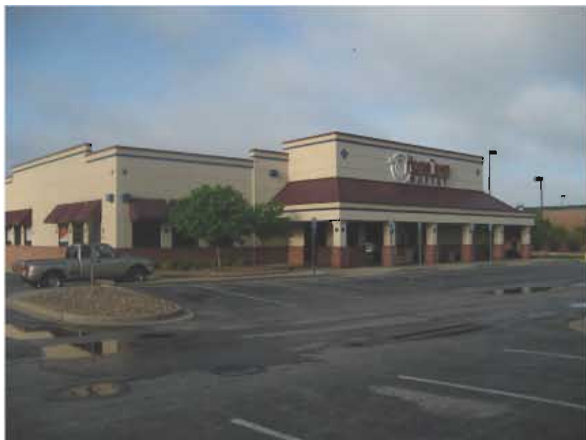
NORTHEAST VIEW OF EXISTING BUILDING
