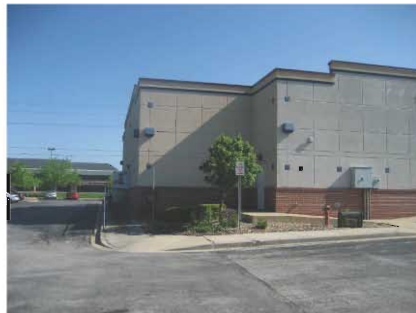
SOUTHWEST VIEW OF EXISTING BUILDING
