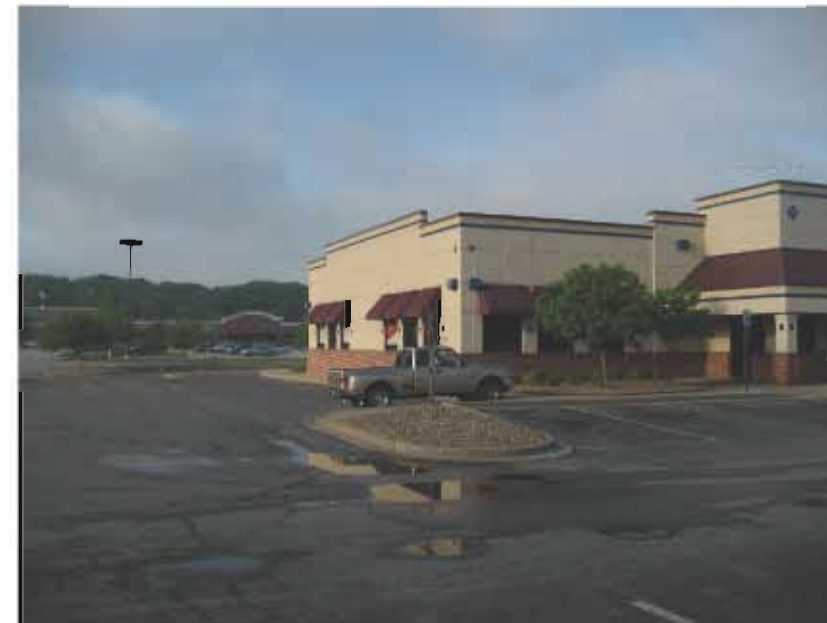
NORTHEAST VIEW OF EXISTING BUILDING
