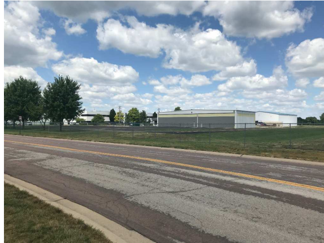
VIEW LOOKING NORTHWEST (SOUTH SIDE OF EDISON)
