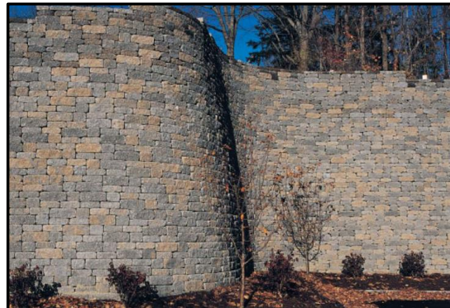
Figure 5: Mosaic Retaining Wall
