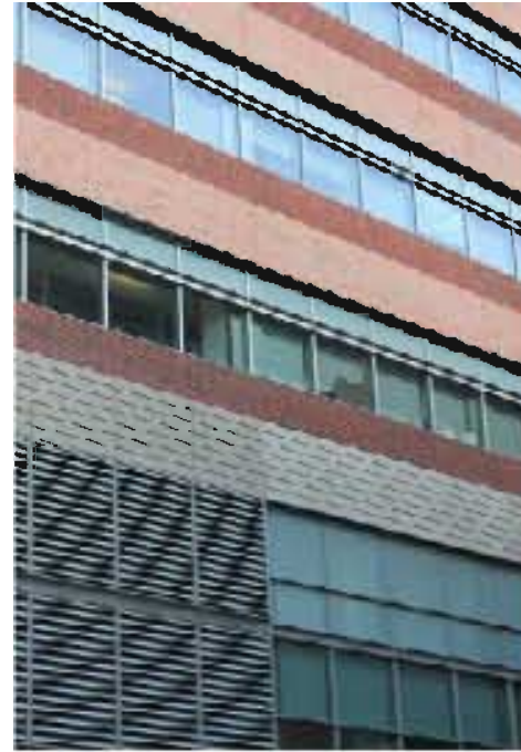
Existing Building CC
