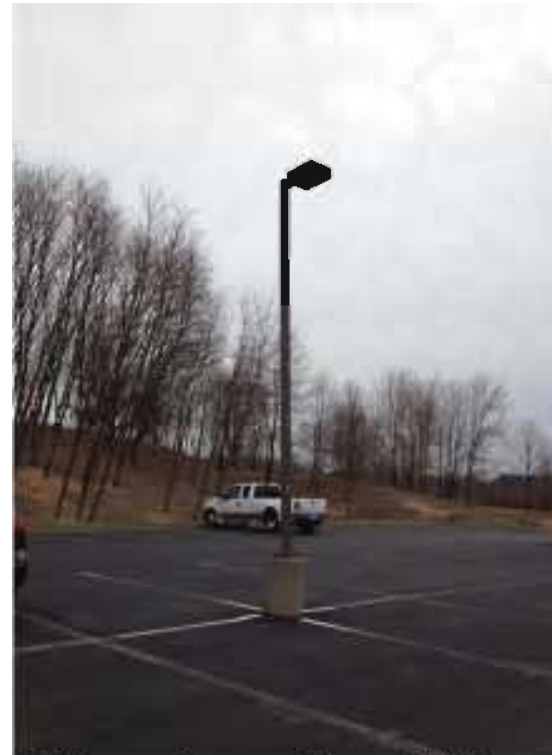
Existing surface parking and hill beyond
