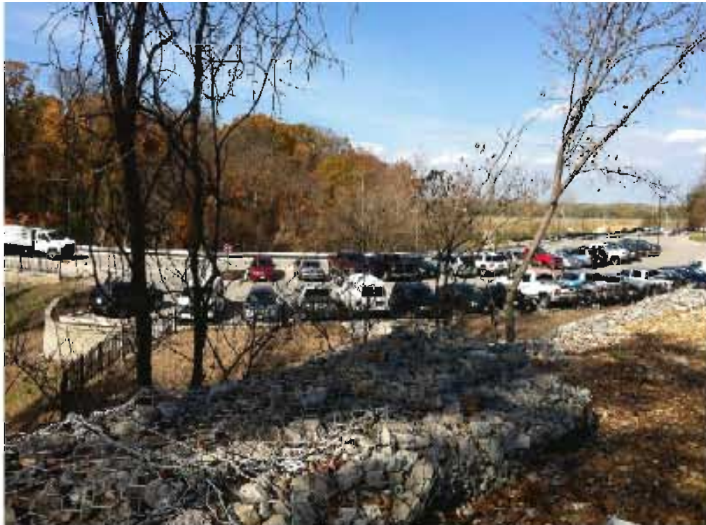
Typical existing gabion wall, and view to farm land beyond
