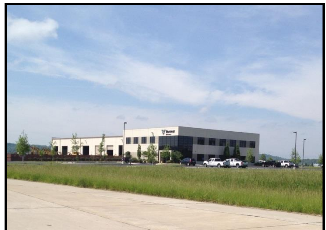
Adjacent property to southwest
