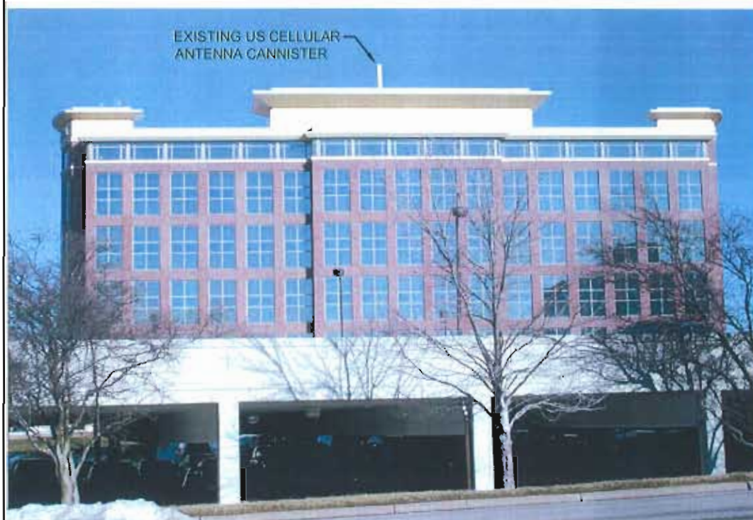
LOOKING EAST EXISTING
