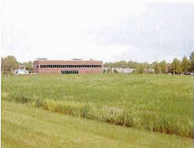
E - VIEW LOOKING NORTHEAST
