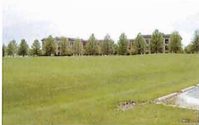
D - VIEW LOOKING SOUTHEAST
