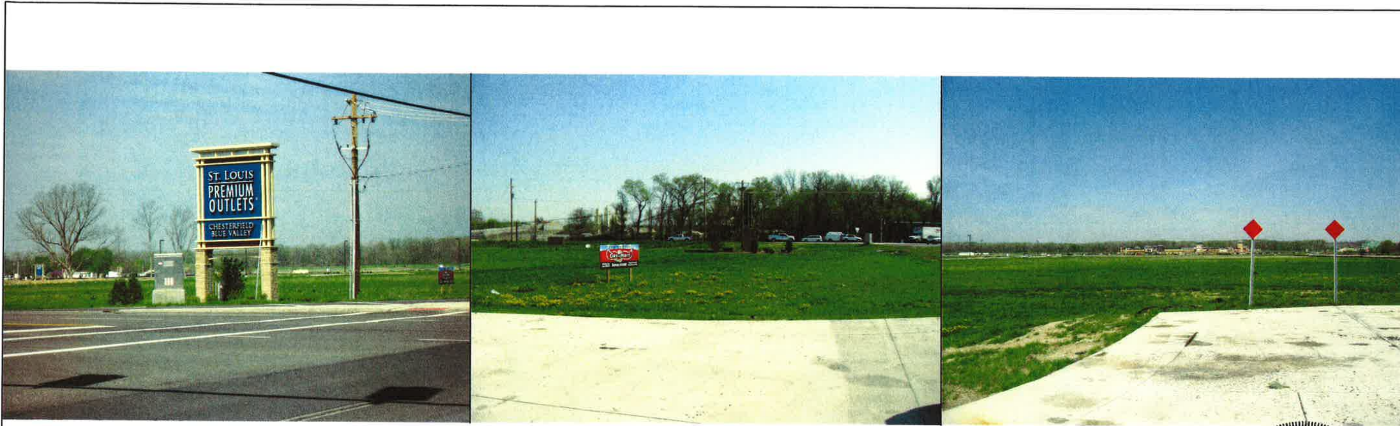
PANORAMIC VIEWS OF EXISTING SITE.
