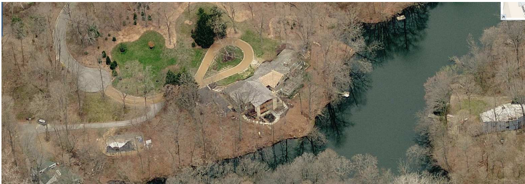
Looking west at existing structure on subject site
