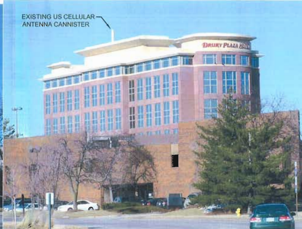
LOOKING NORTHEAST EXISTING
