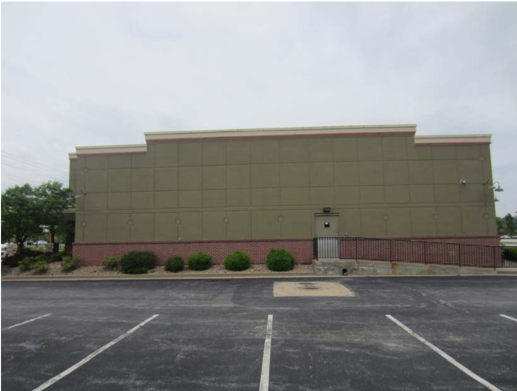
View of existing west façade
