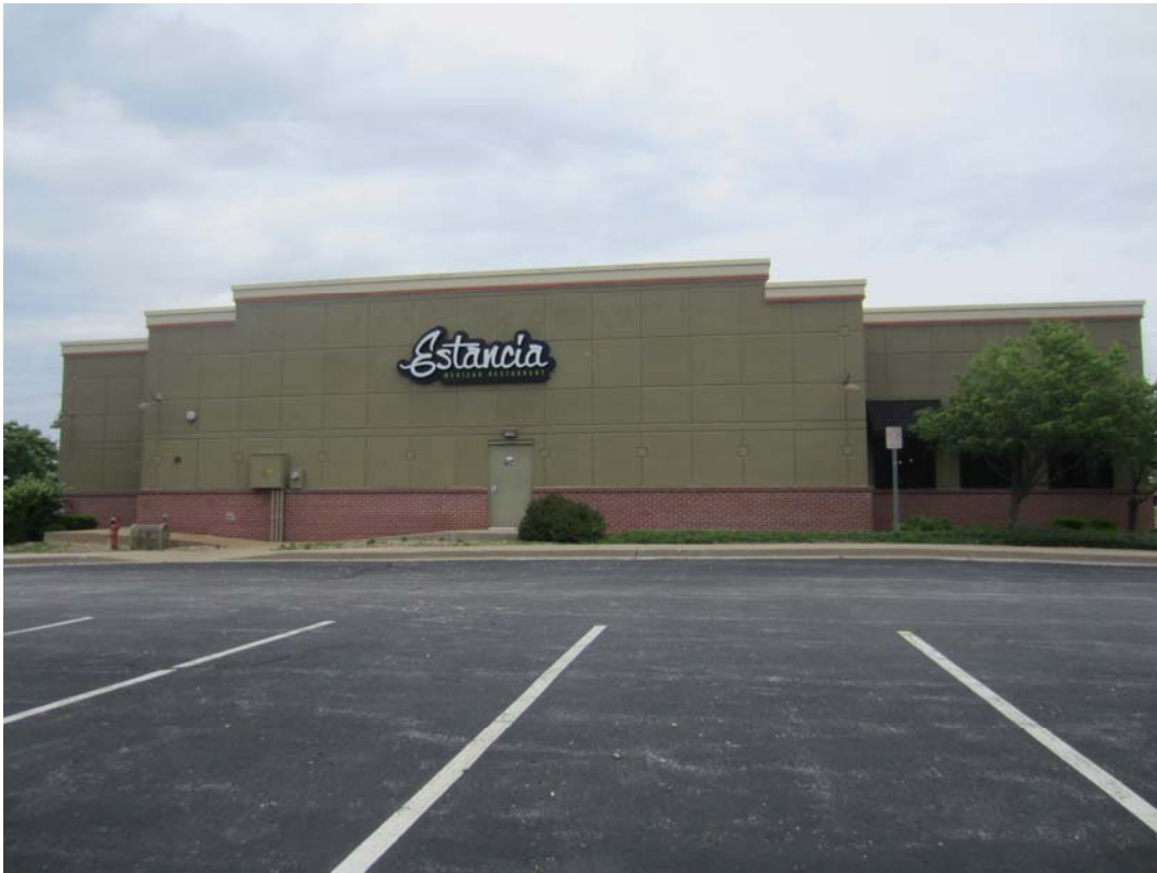
View of existing west façade
