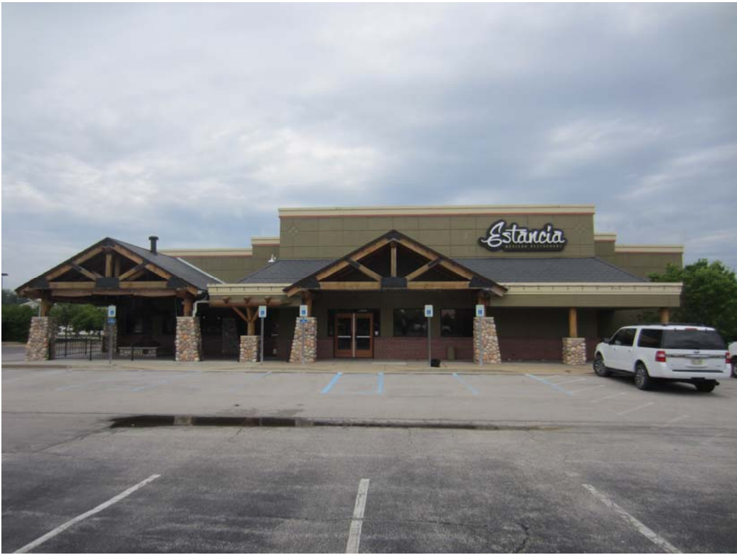
View of existing north façade
