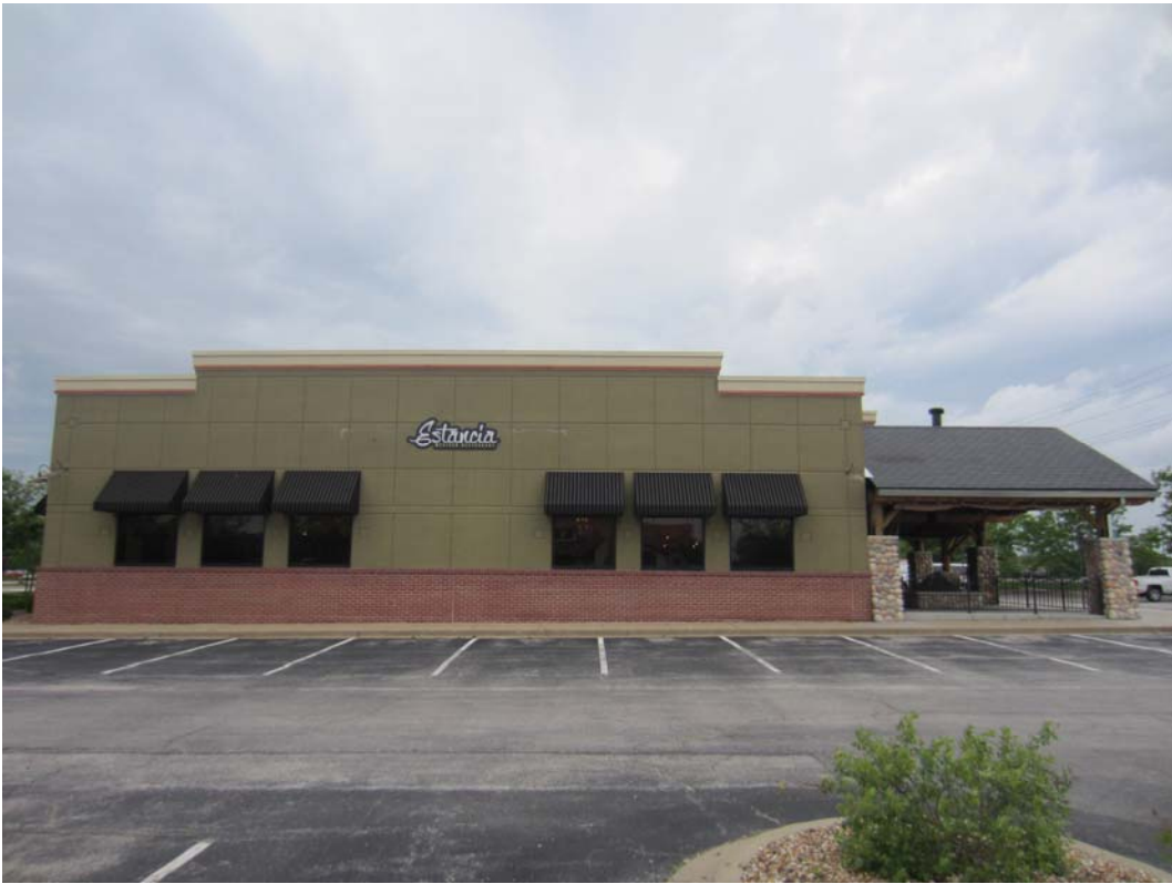
View of existing east façade
