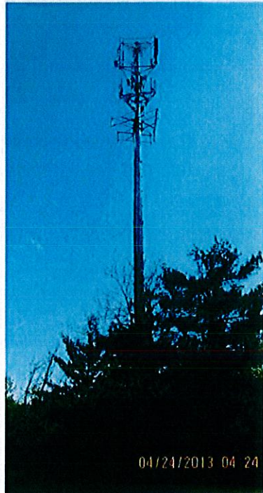
PHOTO OF EXISTING TOWER ELEVATION
