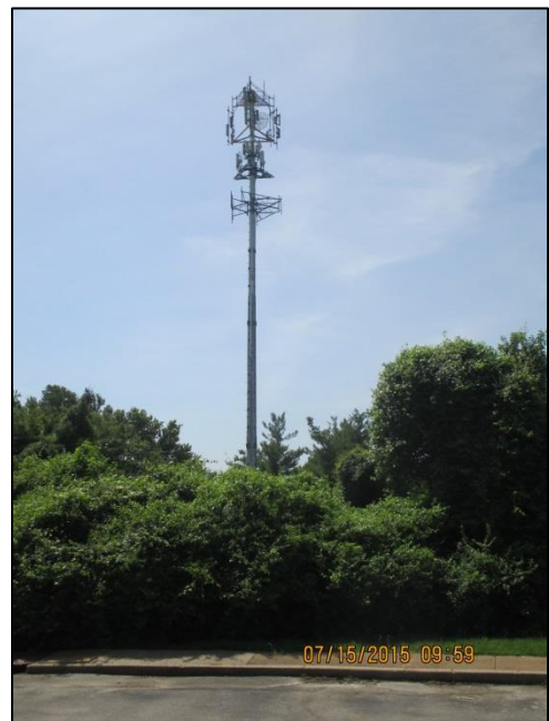
Figure 2: Photo of Tower
