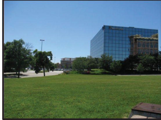
View looking west towards the Chesterfield Mall
