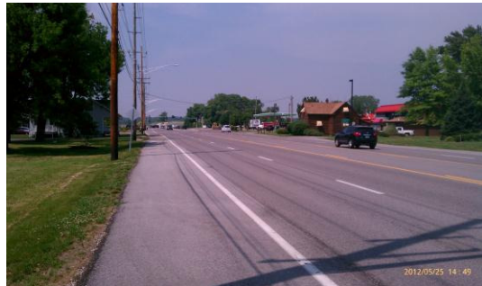
View looking N up Long Rd.
