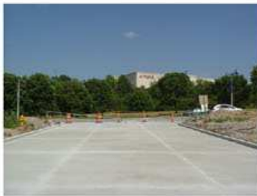
VIEW FROM "B" LOOKING SOUTHWEST
