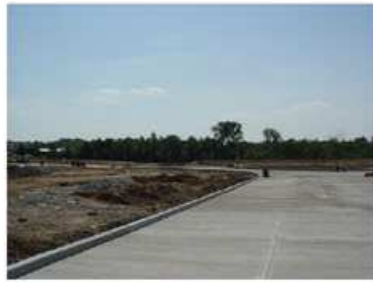
VIEW FROM "B" LOOKING NORTHEAST
