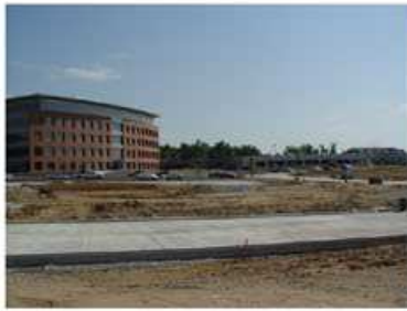
VIEW FROM "A" LOOKING SOUTHEAST
