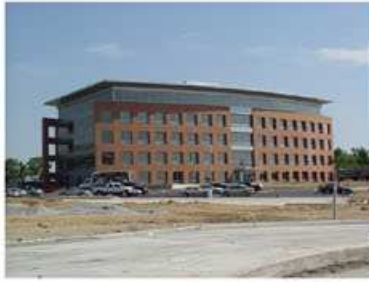
VIEW FROM "C" LOOKING SOUTH
