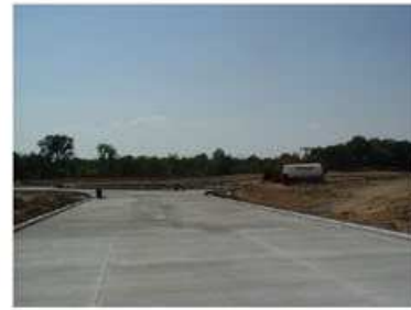
VIEW FROM "B" LOOKING TO ROUNDABOUT
