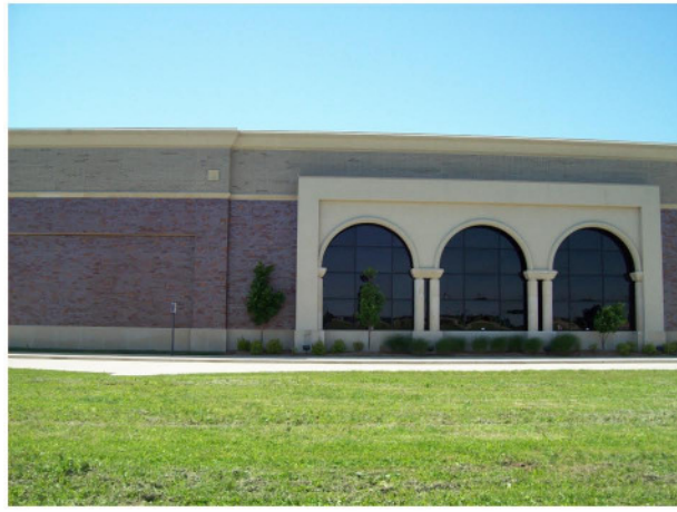
VIEW LOOKING WEST FROM "C"
