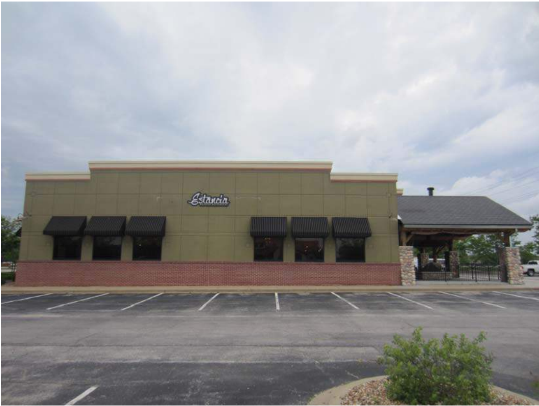
View of existing east façade
