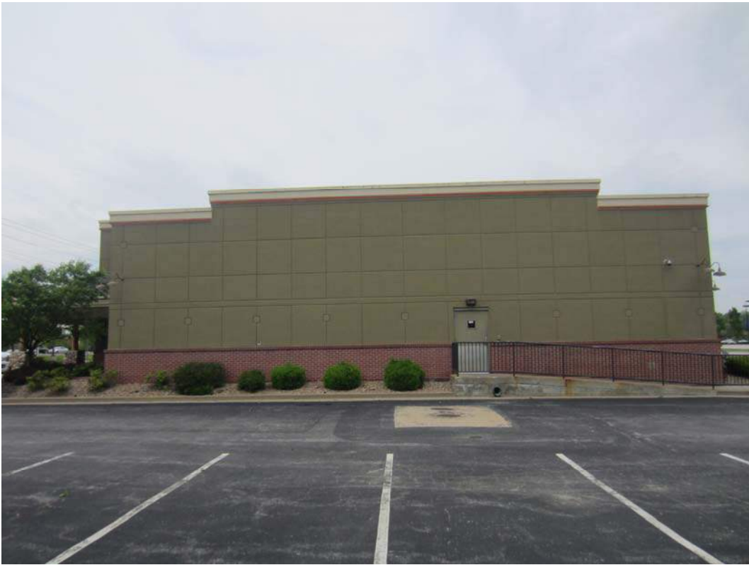
View of existing west façade
