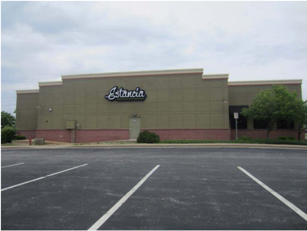
View of existing west façade
