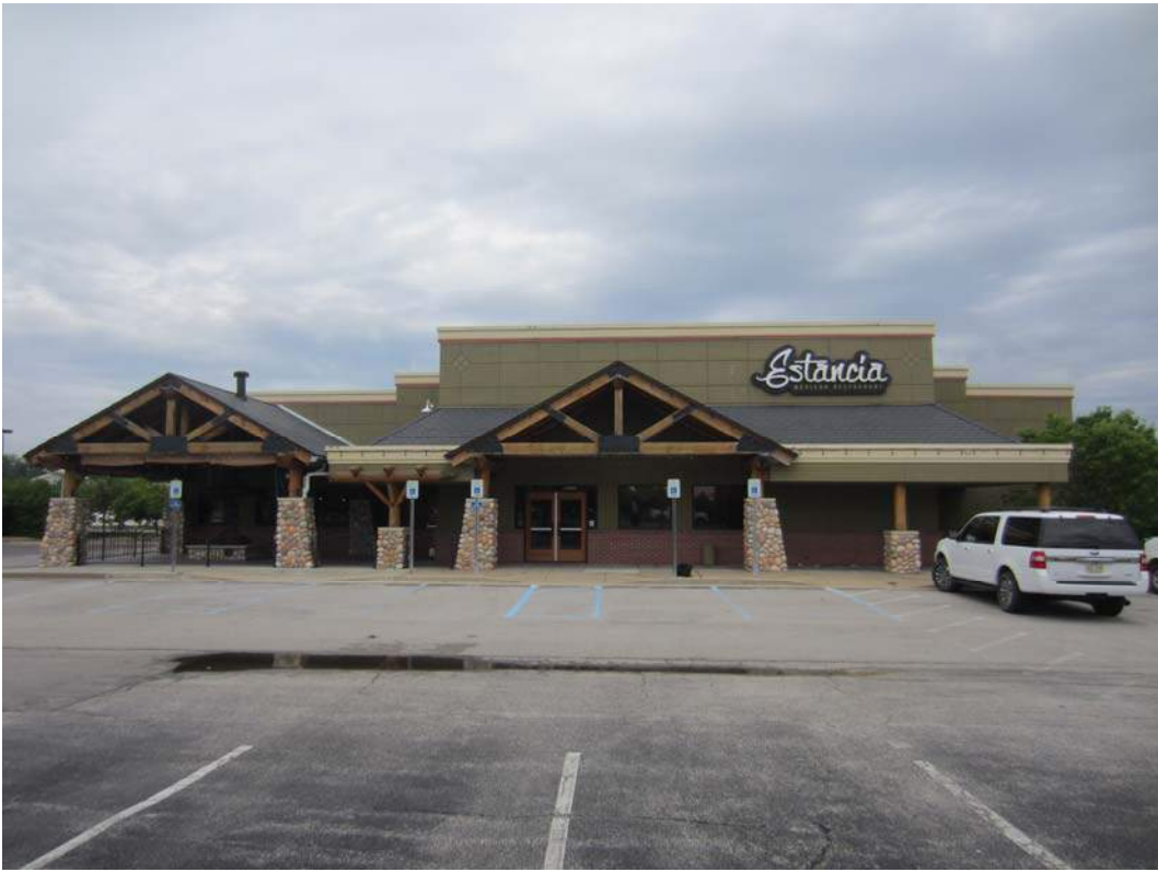
View of existing north façade
