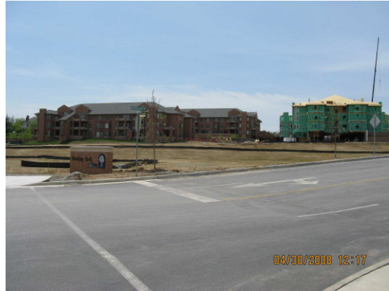
View looking southwest from Woods Mill Road
