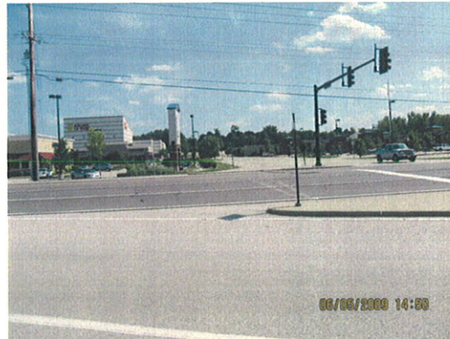
Looking south across Chesterfield Airport Road
