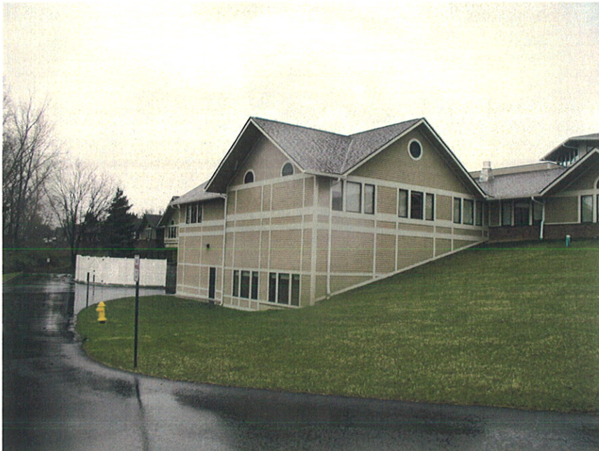
View of western elevation
