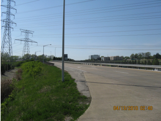
View looking west along S. Outer 40 Road
