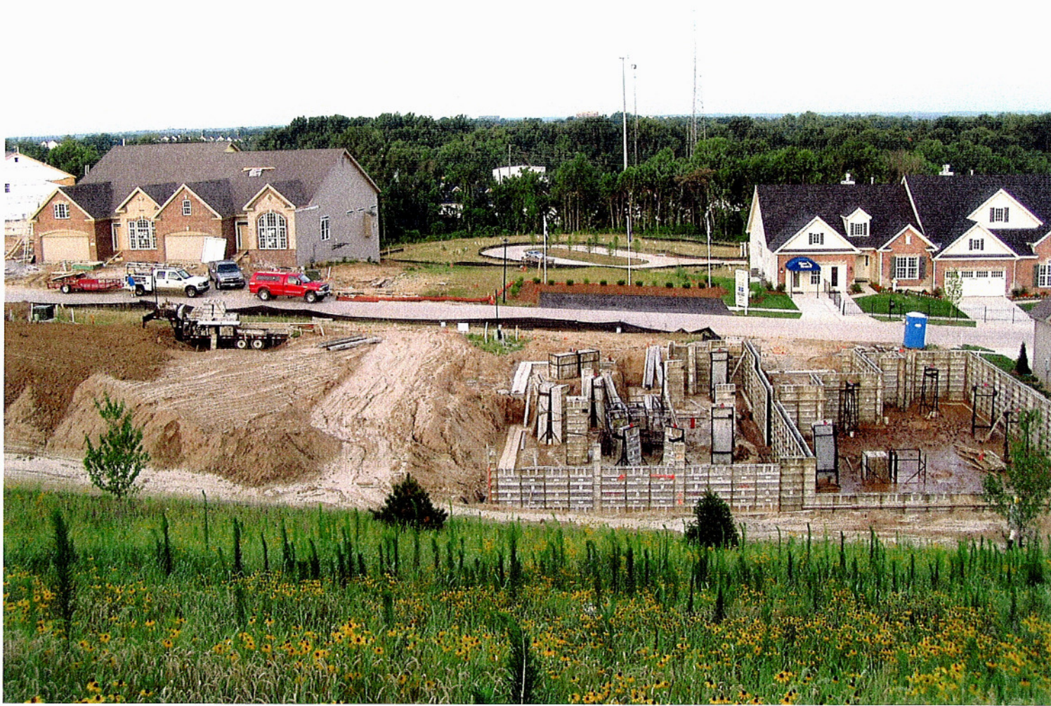
Neighbor to South – Kendall Place
