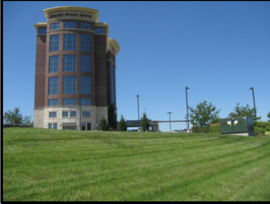
View looking north from inside the undeveloped lot.
