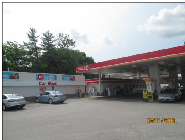
Figure 2: Carwash, Convenience Store, and Gas Canopy
