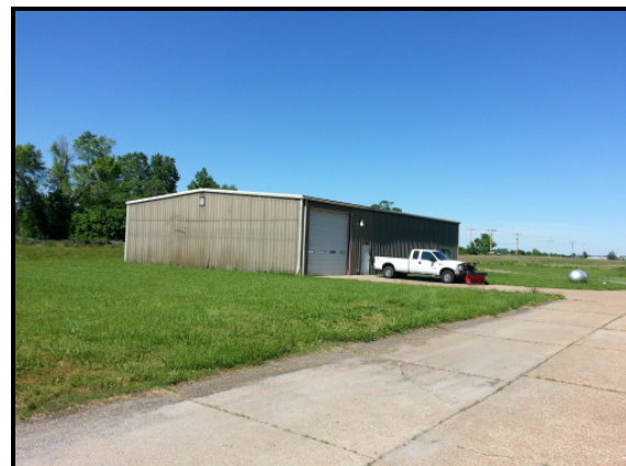
Existing metal building on site
