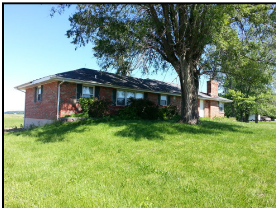
Existing residential structure on site
