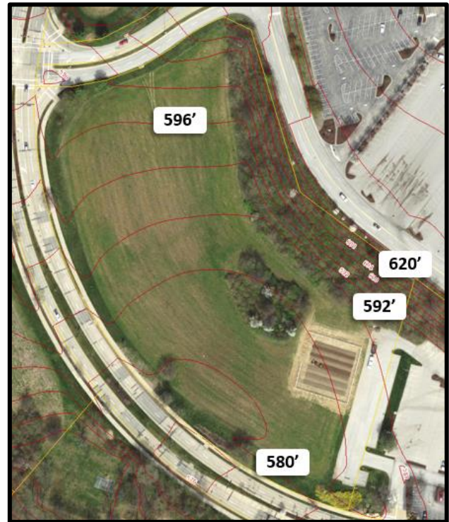
Figure 8: Current Site Grade
