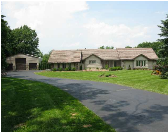
Looking northwest at existing structure on subject site
