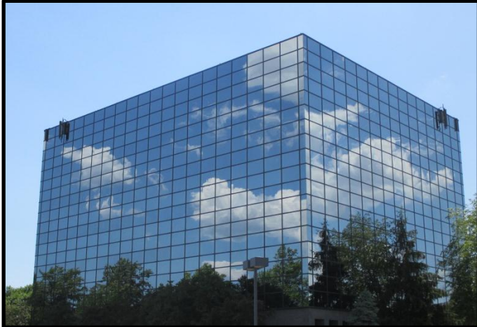
Figure 2. Site Photo – North and East Facades
