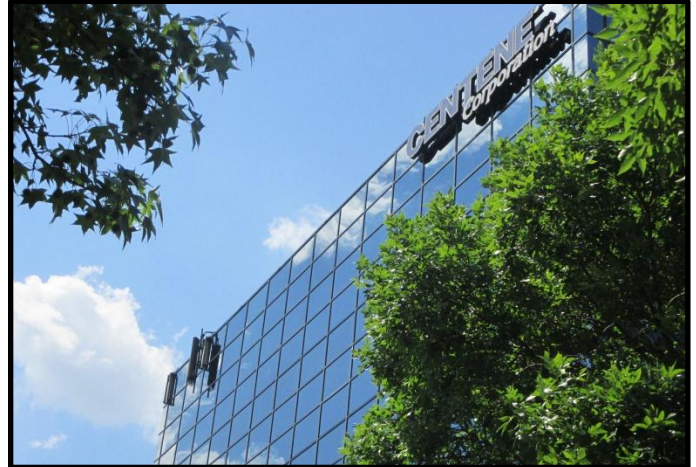
Figure 3. Site Photo – South Facade
