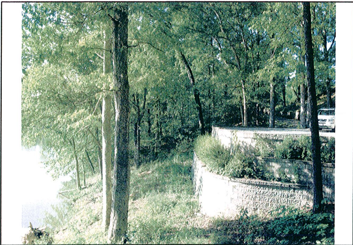
VIEW OF RETAINING WALLS AT EXISTING DRIVEWAY TURNAROUND
