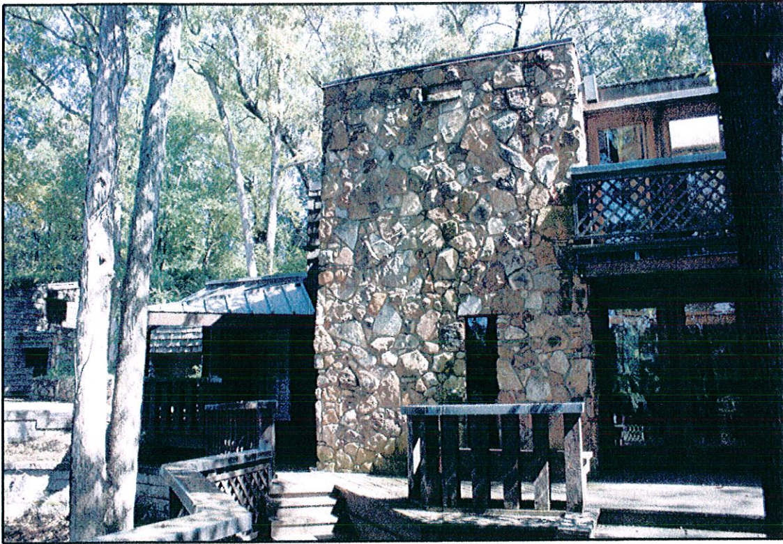
EXISTING HOUSE TO BE DEMOLISHED
