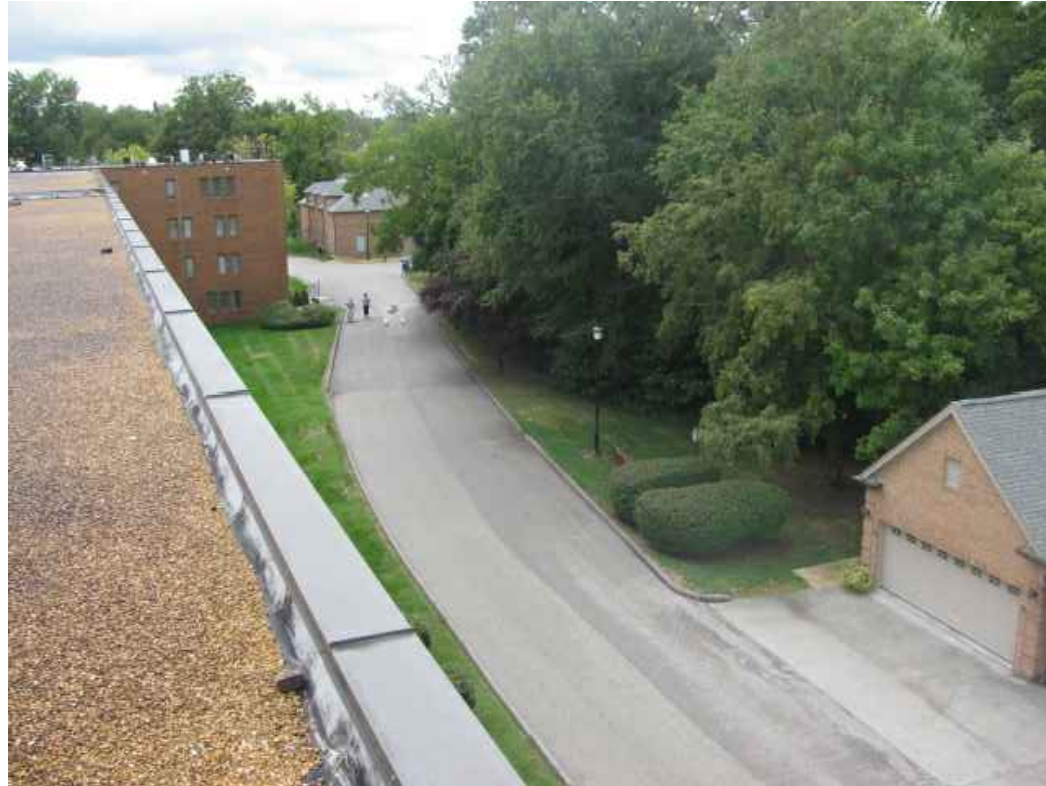
DRIVE AND MAINTENANCE BUILDING
