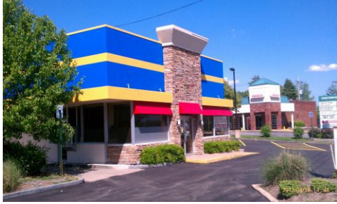
View of the front of the Structure
