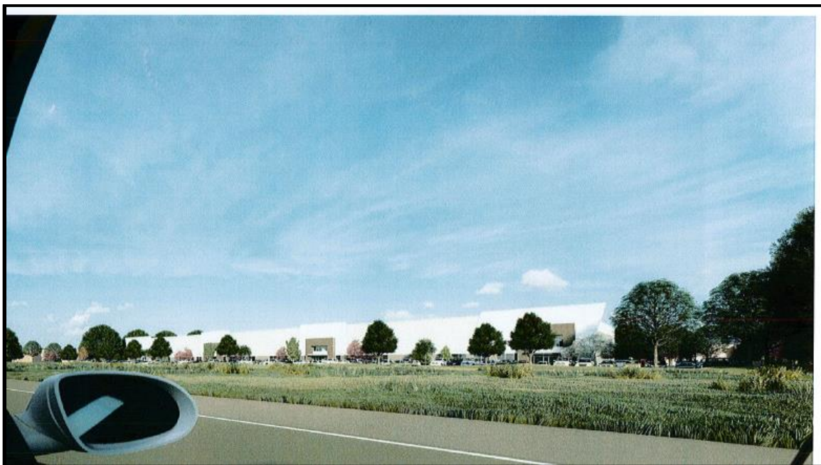
Figure 5: North Elevation as seen by vehicles traveling east on I-64.
