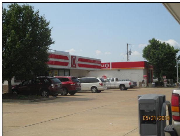
Figure 2: Convenience Store & Carwash
