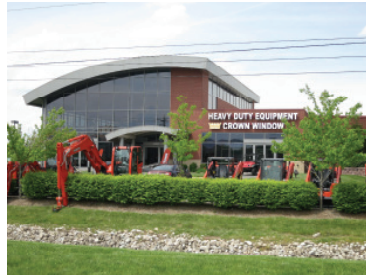
E - VIEW LOOKING NORTH (EXISTING BUILDING)
