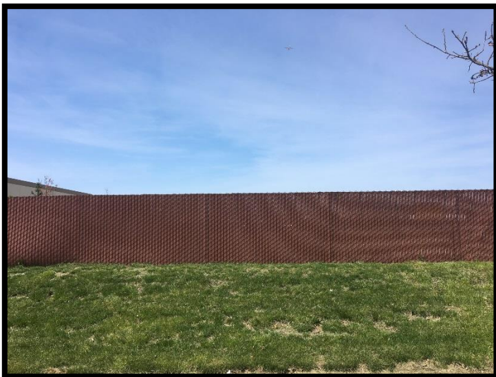
Figure 3: Existing Fencing Material
